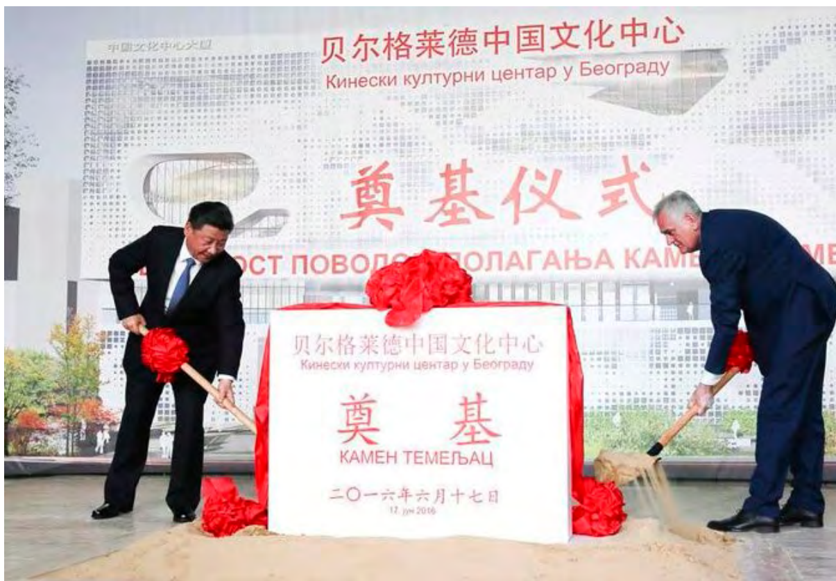
Figure 4: Xi Jinping and Tomislav Nikolić, Presidents of China and Serbia, laying the foundations of the Chinese Cultural Centre in Belgrade, June 2016
